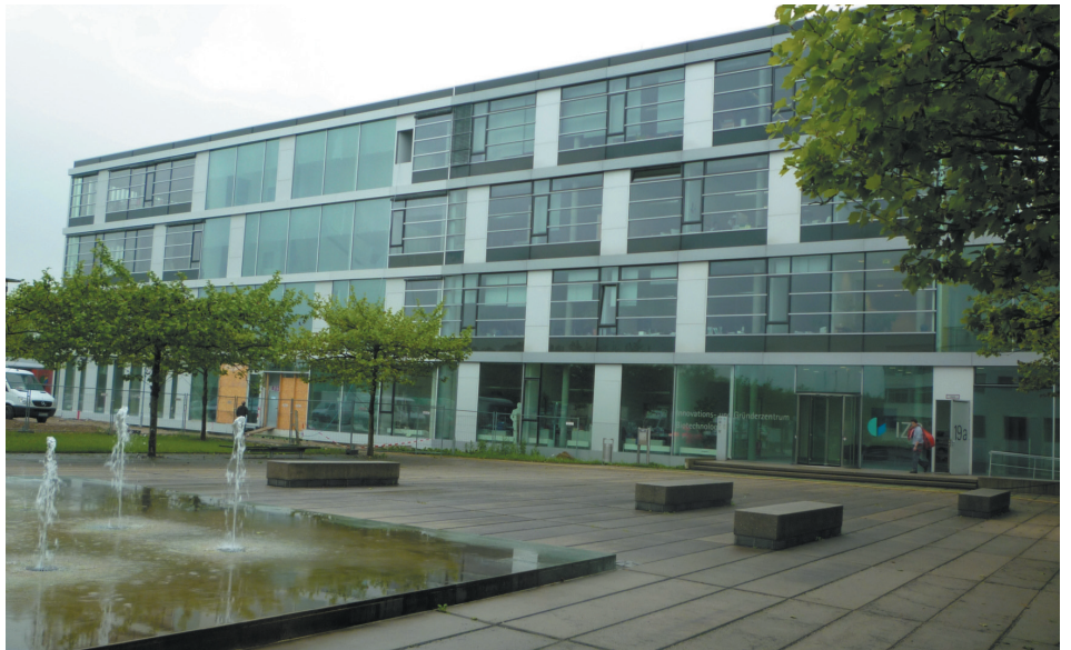
IZB Martinsried West 2 building: completion due in September
